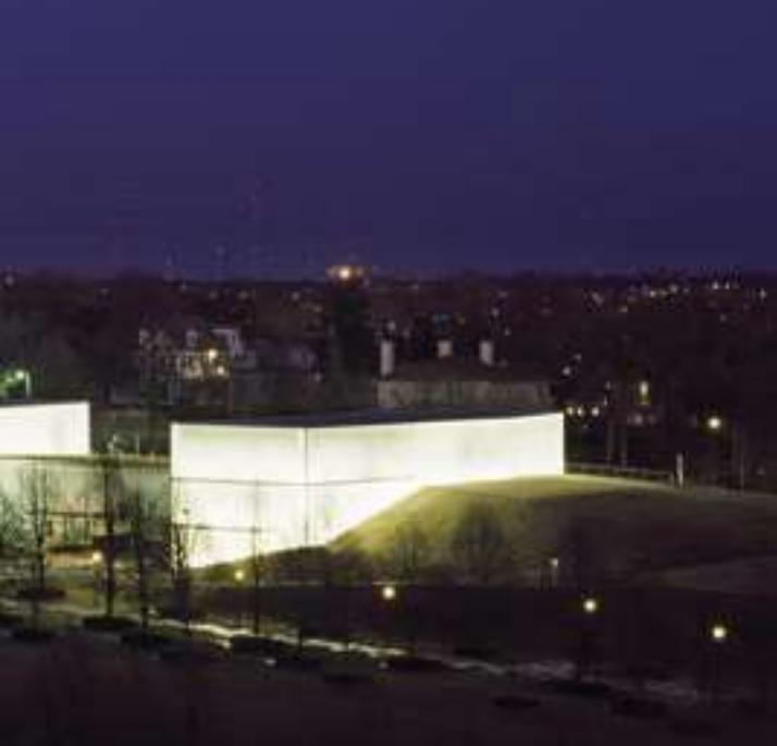
The lenses are instruments of light, gathering and diffusing natural light to the interior during the day and glowing in the sculpture park at night. The lenses' multiple layers of translucent glass gather, diffuse and refract light, at times materializing light like blocks of ice. During the day the lenses inject varying qualities of light into the galleries, while at night the sculpture garden glows with their internal light.
