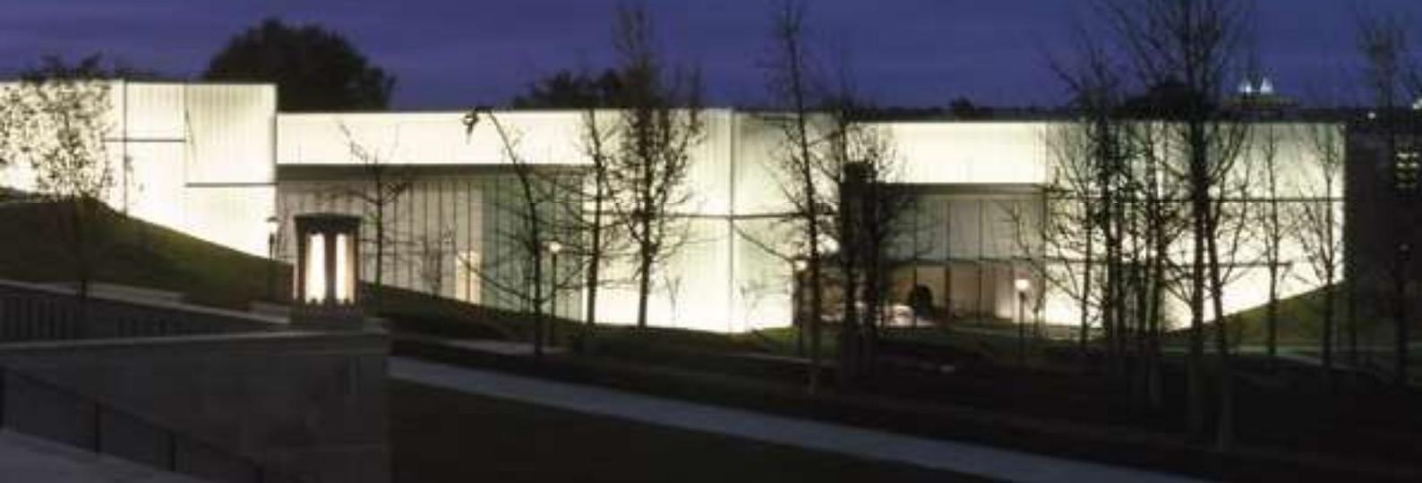
Owing to a solar texture on the outer surface of the channel glass and the sandblasted inner face of this outer wall, the exterior takes on an opalescent sheen in sunlight, rather like chantung silk. Although it sometimes appears flat in even light, as exterior conditions change, a glinting moiré pattern emerges.
